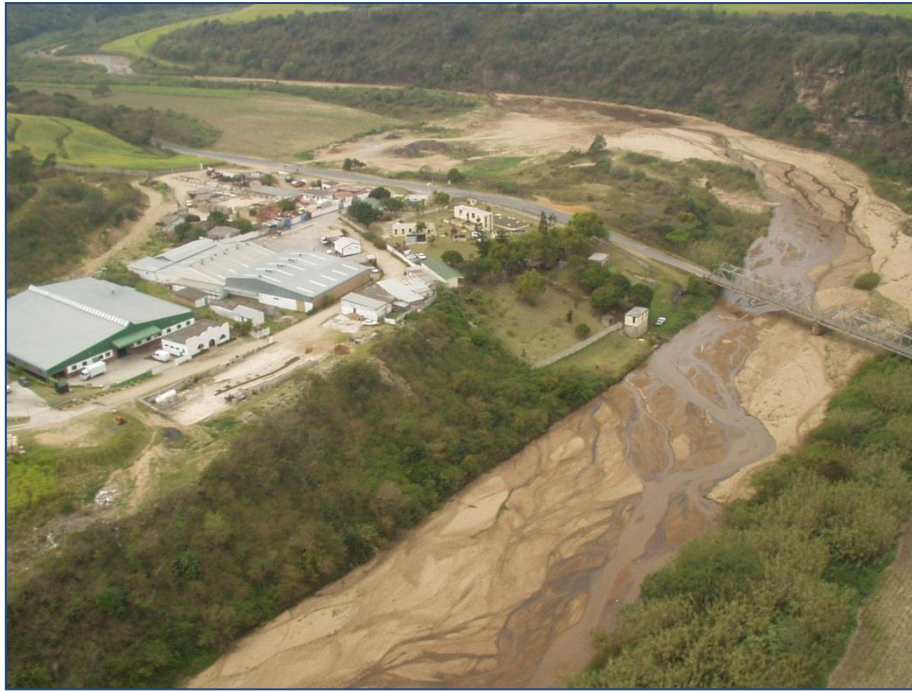
Figure 11.28 Mtwalume Water Treatment Plant.
