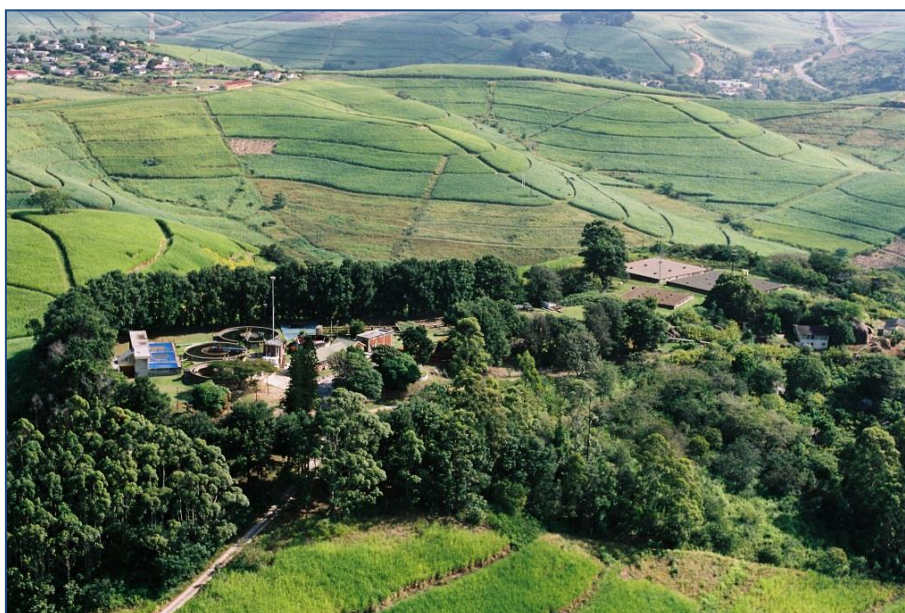
Figure 11.26 Umzinto Water Treatment Plant.
