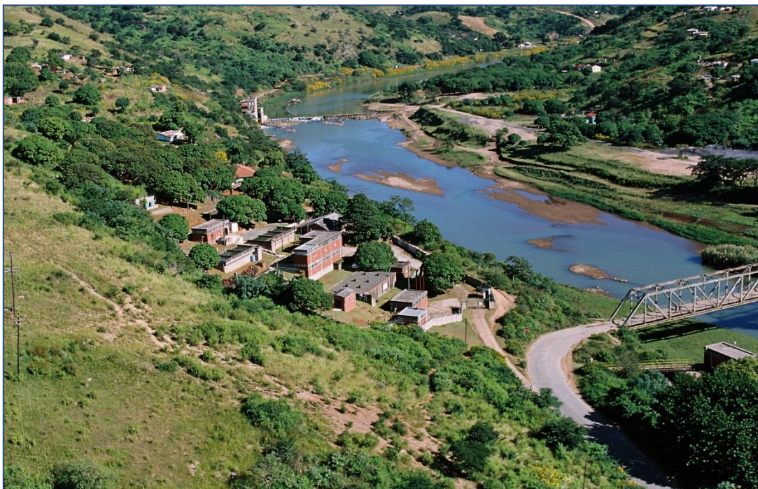
Figure 11.25 Craigieburn Water Treatment Plant (decommissioned).
