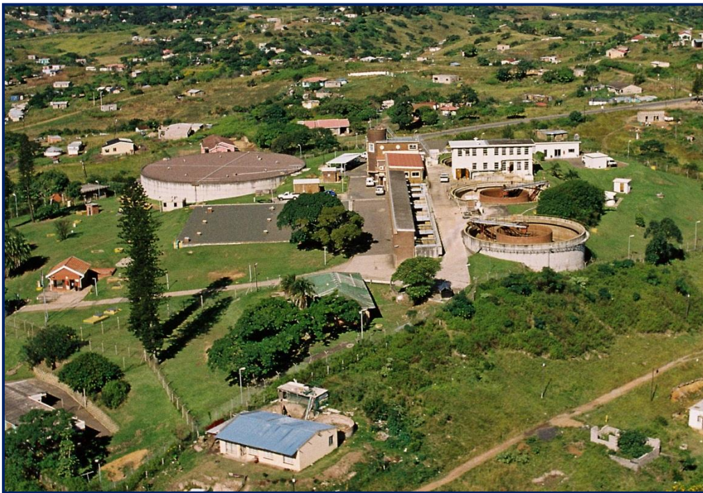
Figure 11.23 Amanzimtoti Water Treatment Plant.
