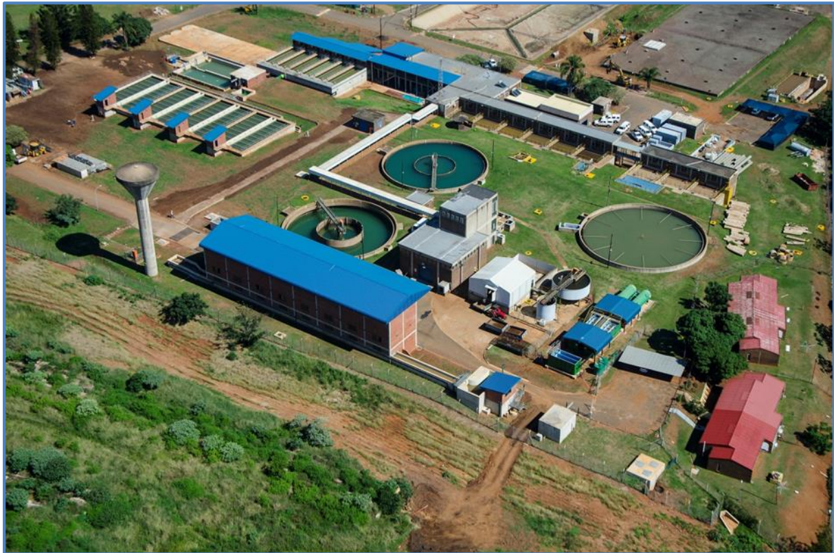
Figure 12.18 Hazelmere Water Treatment Plant.
