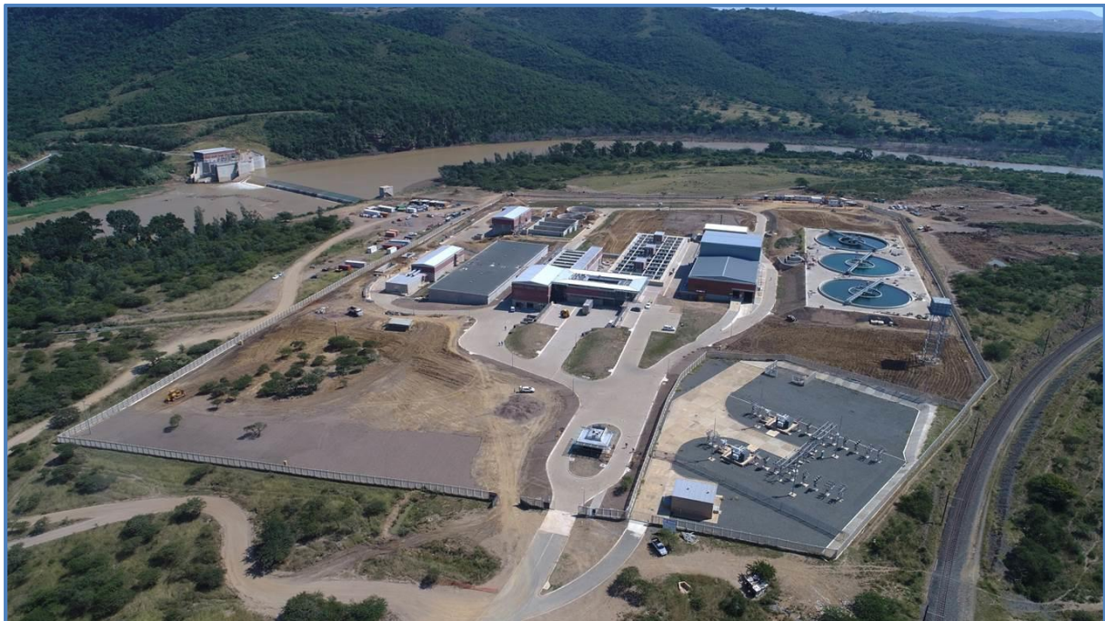
Figure 12.20 Lower Thukela Water Treatment Plant
