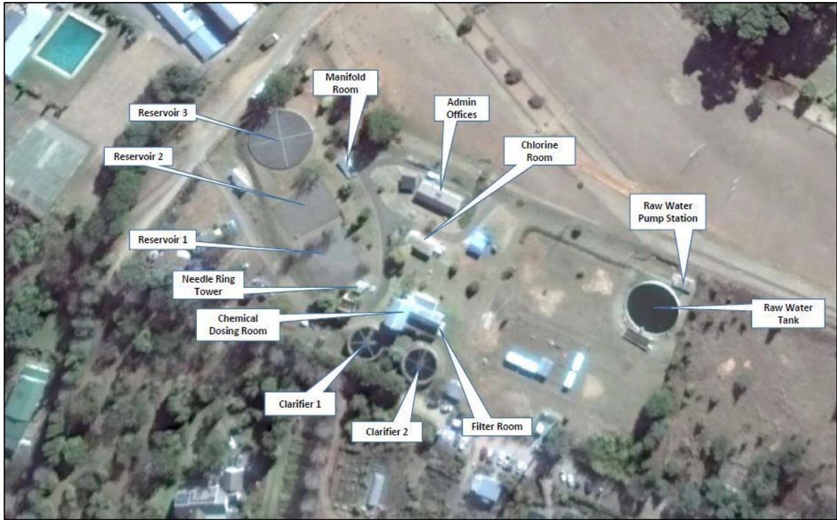
Figure 12.26 Aerial view of the Greytown Water Treatment Plant (Google Earth 2018).
