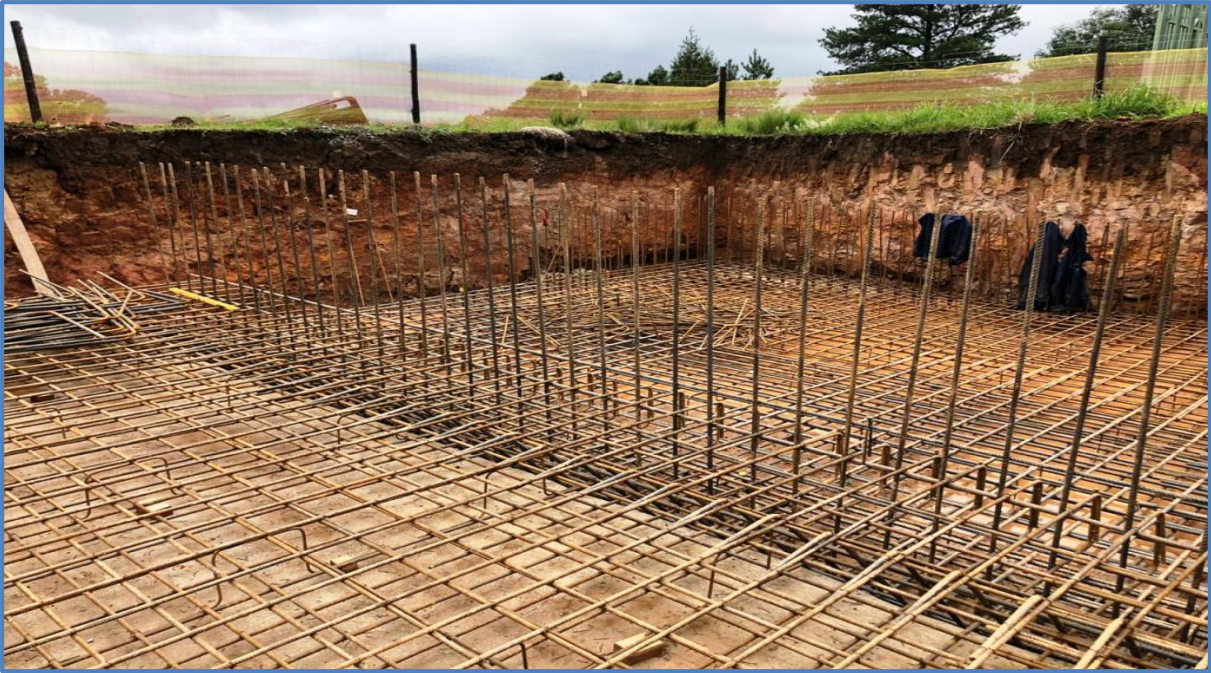
Figure.12.46 Transfer Pump Station in Construction (Late 2019)
