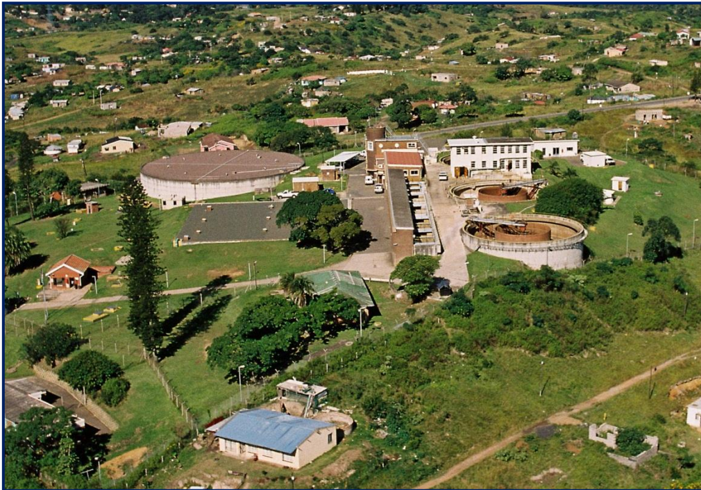
Figure 11.25 Amanzimtoti Water Treatment Plant.
