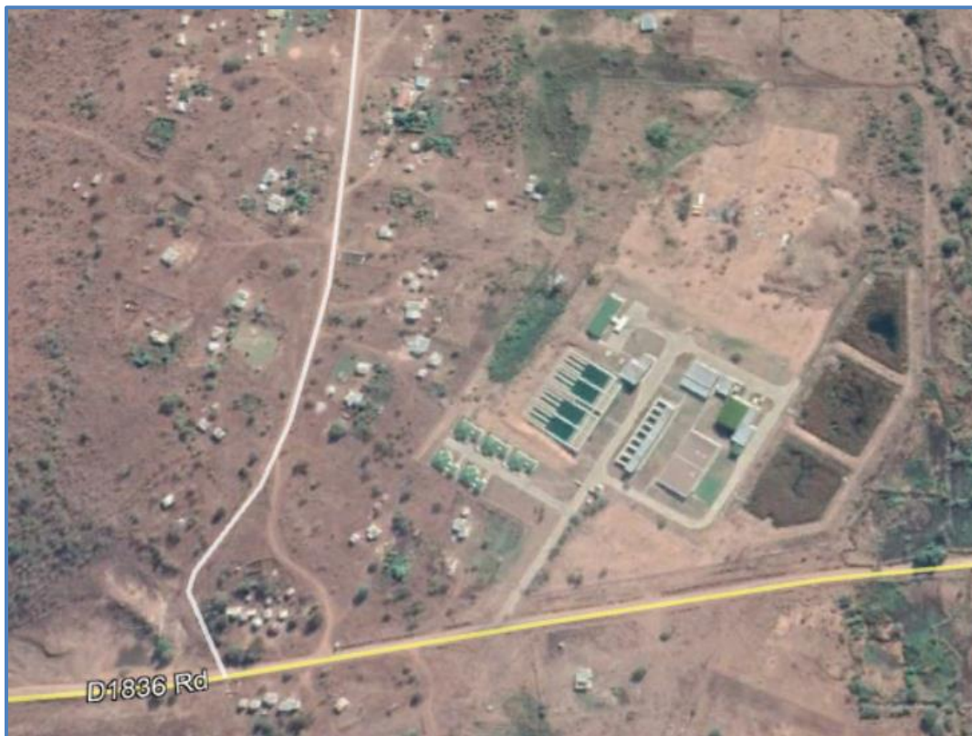
Figure 17.76 Aerial view of Regional Water Treatment Plant (NEW)
