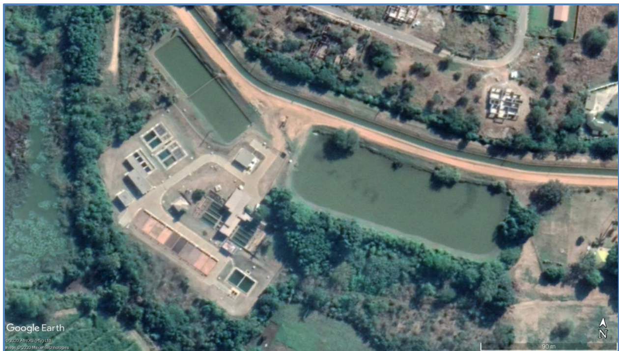
Figure 17.59 Aerial view of Phongola Water Treatment Plant
