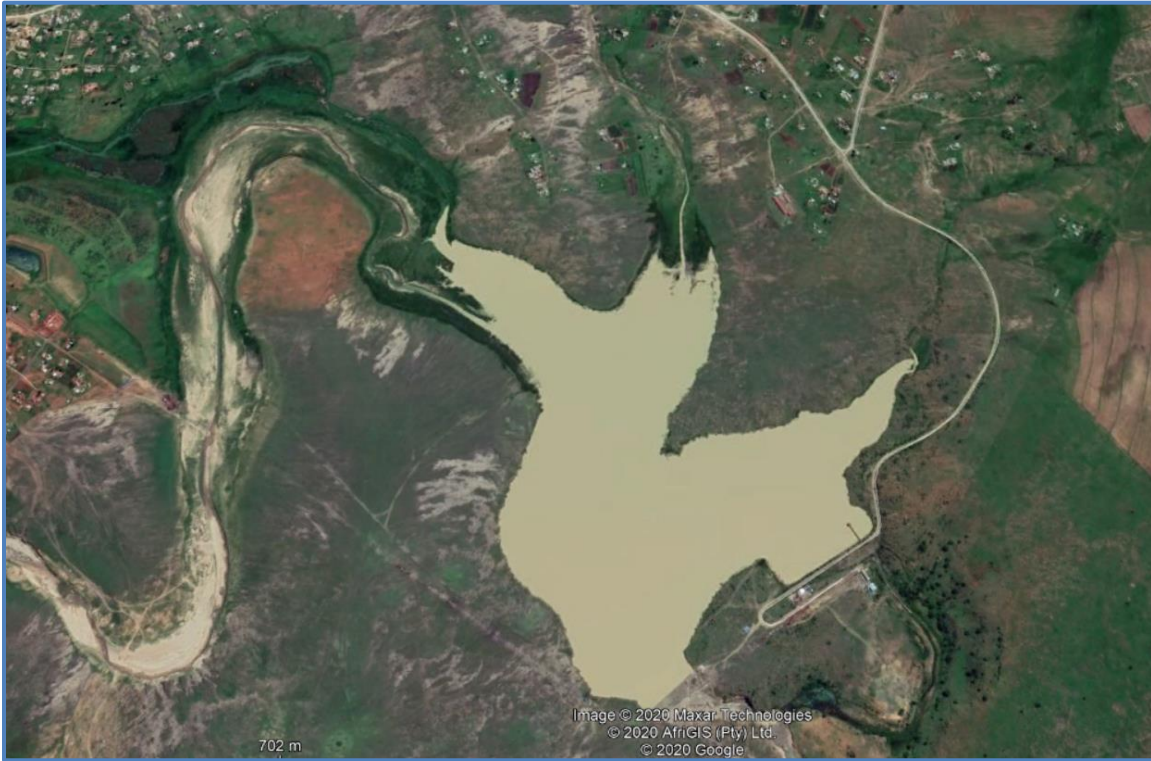
Figure 17.10 Mvunyana Dam (Goole Photo: 2020)
