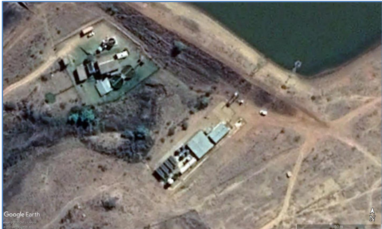
Figure 17.55 Aerial view of Belgrade Water Treatment Plant
