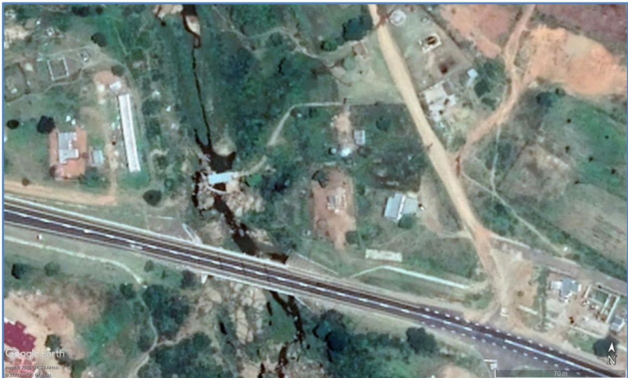
Figure 17.57 Aerial view of Spekboom Water Treatment Plant
