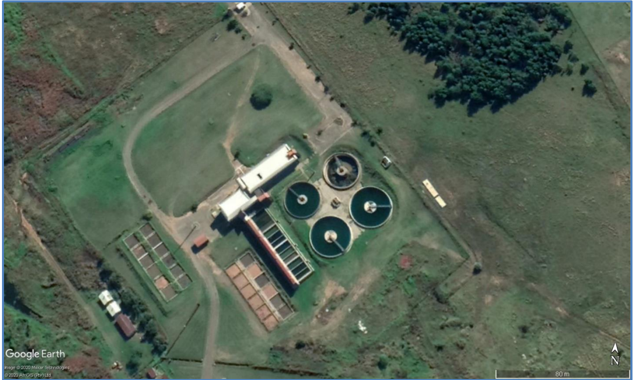
Figure 17.27 An Aerial view of the Klipfontein WTP
