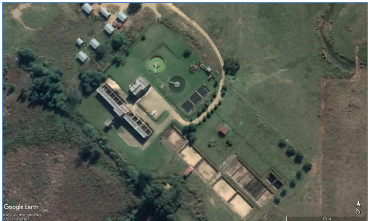
Figure 17.26 An Aerial view of the Bloemveld WTP
