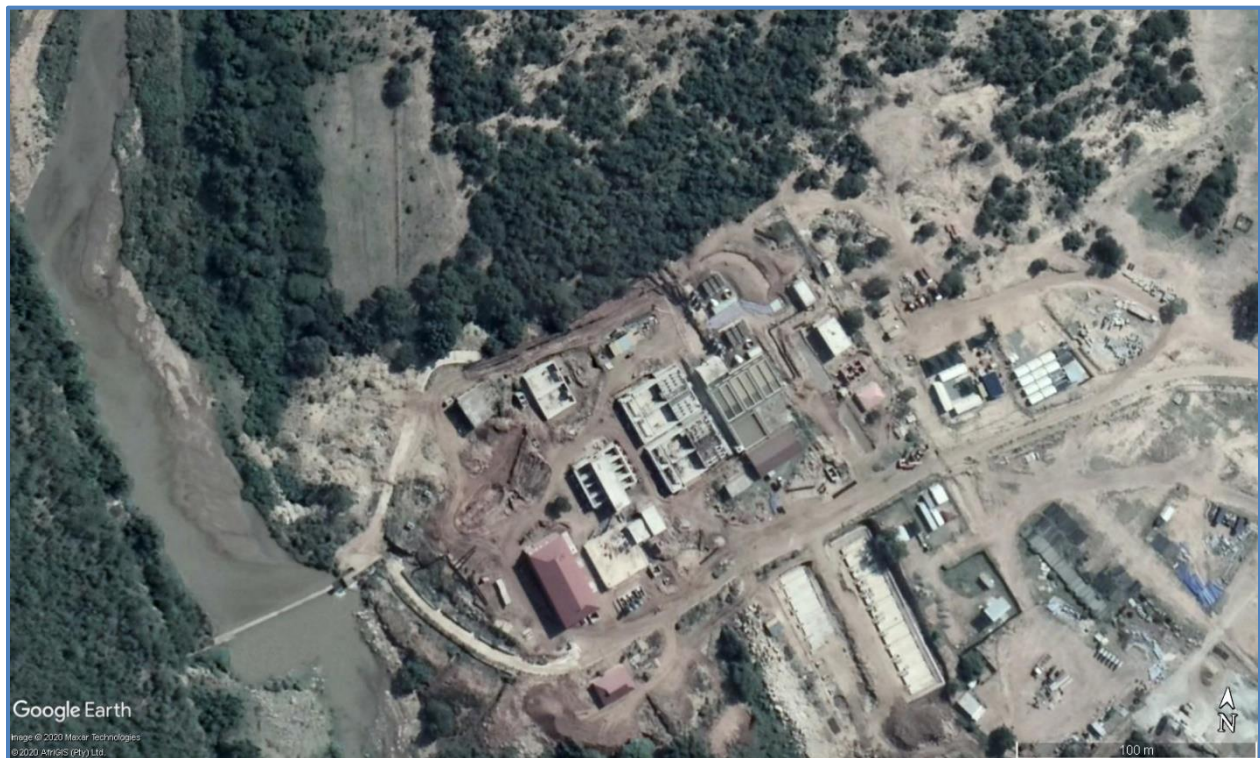
Figure 17.24 An Aerial view of the Usuthu WTP
