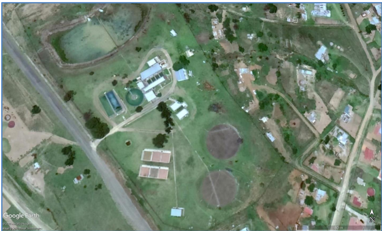
Figure 17.29 An Aerial view of the Mondlo WTP
