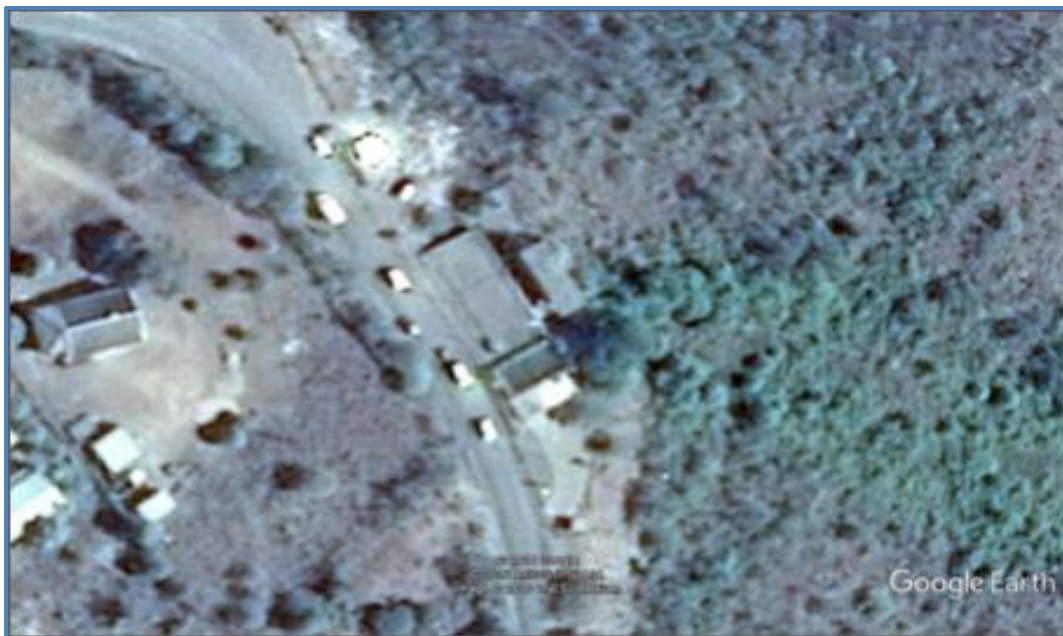
Figure 17.67 Aerial view of Jozini Old Water Treatment Plant
