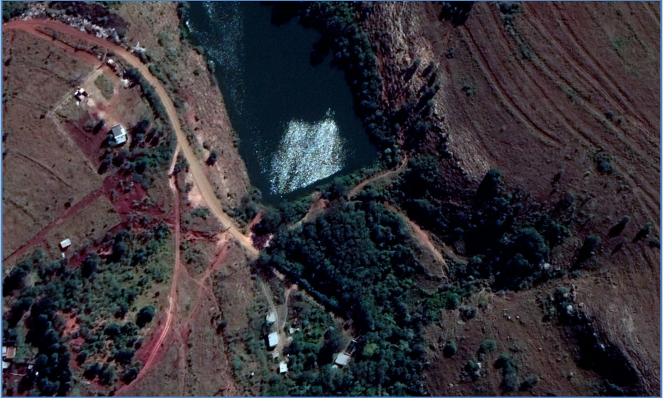
Figure 17.20 An Aerial view of the Embile WTP and the Embile Dam
