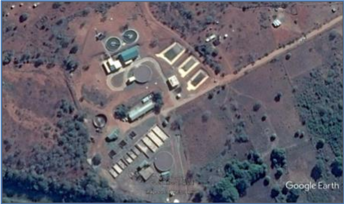
Figure 17.73 Aerial view of Shemula New Water Treatment Plant
