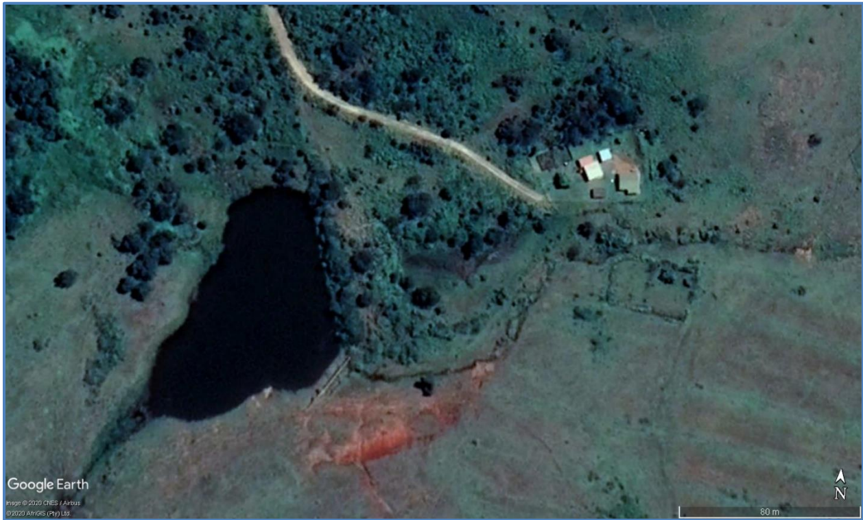
Figure 17.17 Aerial view of the Nkonjeni Dam and Nkonjeni Water Treatment Plant
