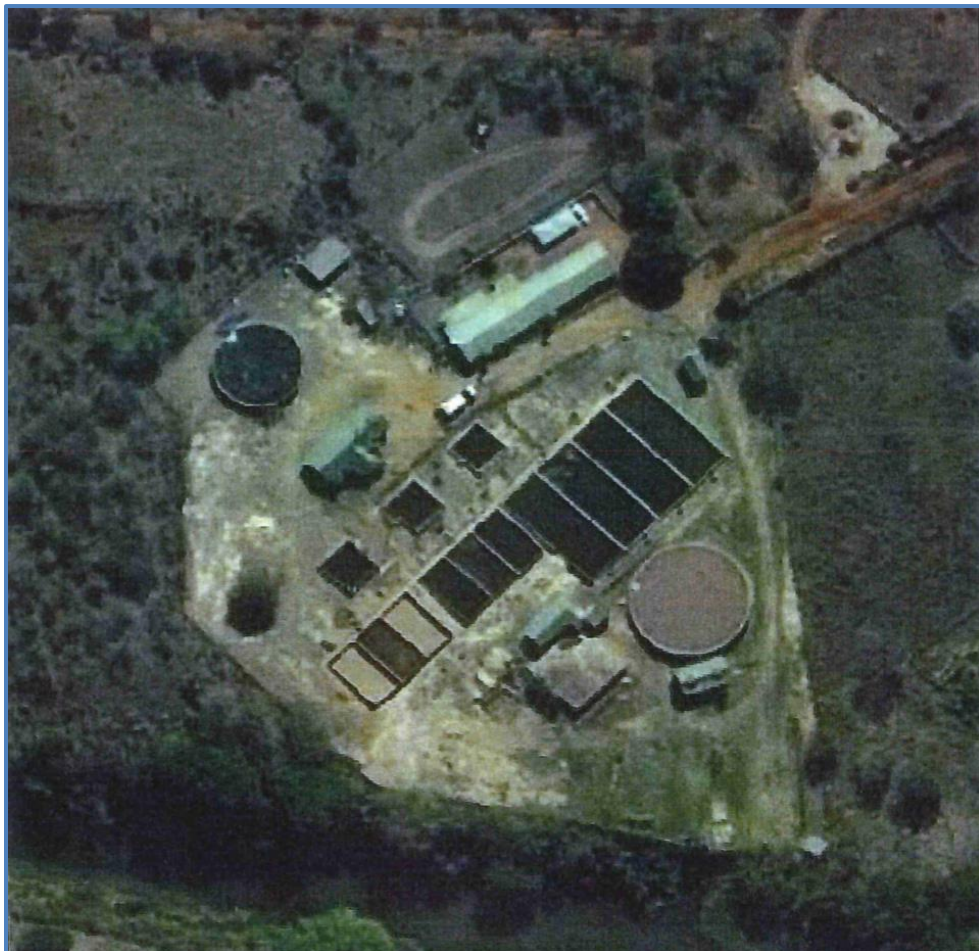
Figure 17.72 Aerial view of the Shemula (Old) WTP
