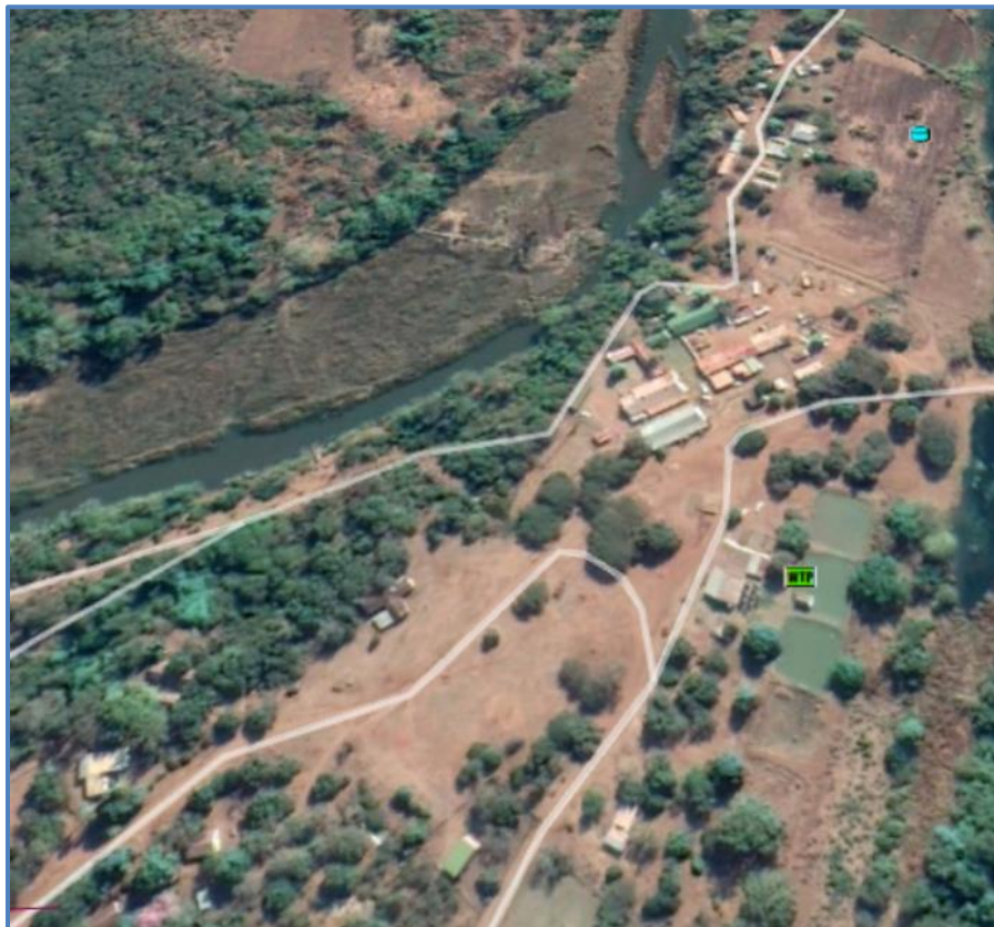
Figure 17.61 Aerial view of Mjindi Water Treatment Plant
