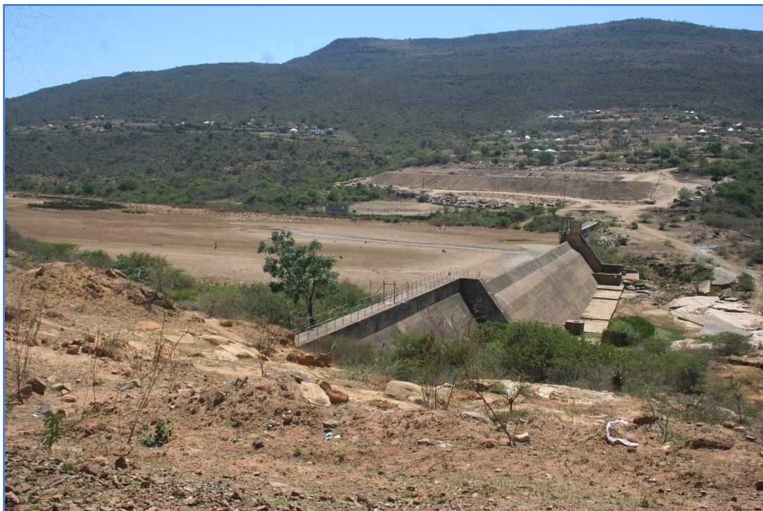
Figure 17.8 Vuna Dam (The Siyasiza Trust Facebook Photo upload: 2015)
