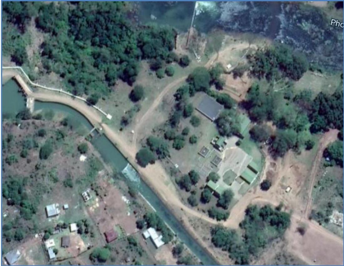
Figure 17.68 Aerial view of Jozini New Water Treatment Plant
