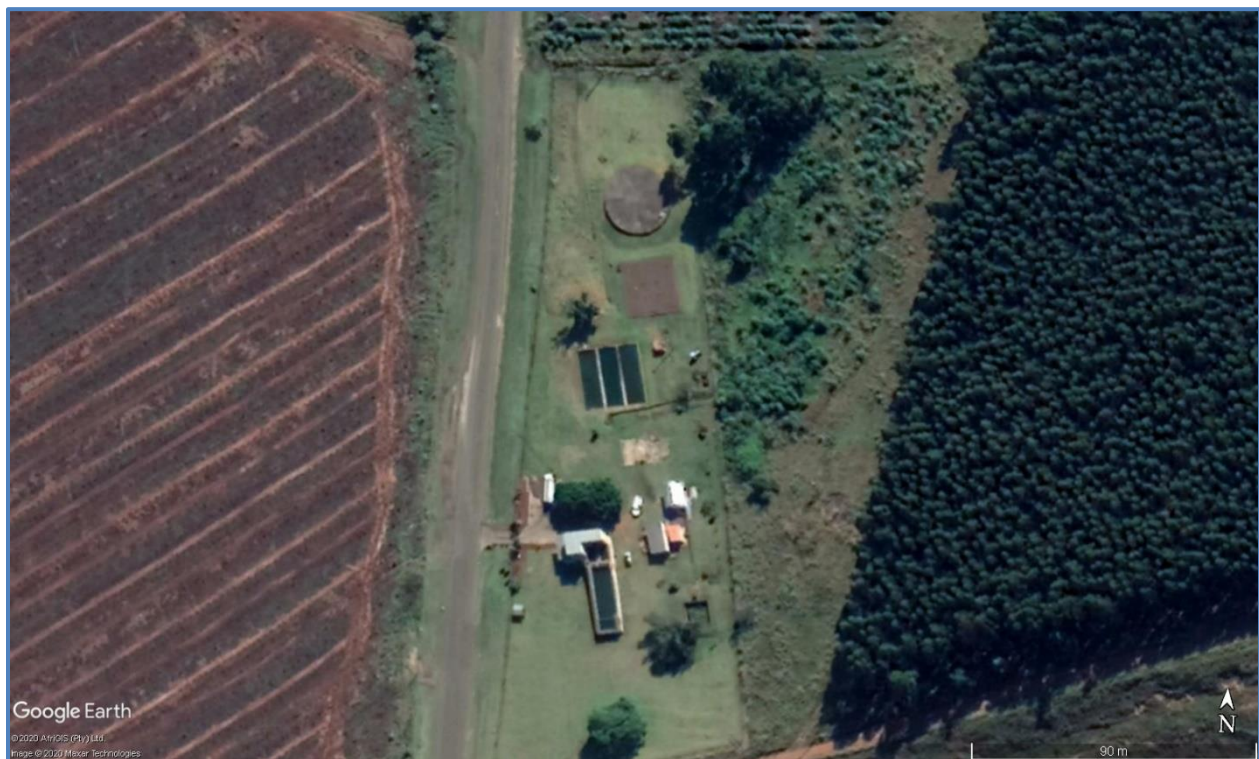
Figure 17.51 Aerial view of Edumbe Water Treatment Plant
