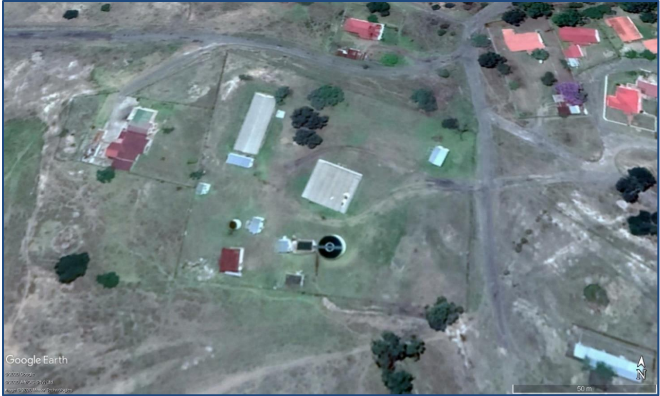
Figure 17.48 Aerial view of Coronation WTP
