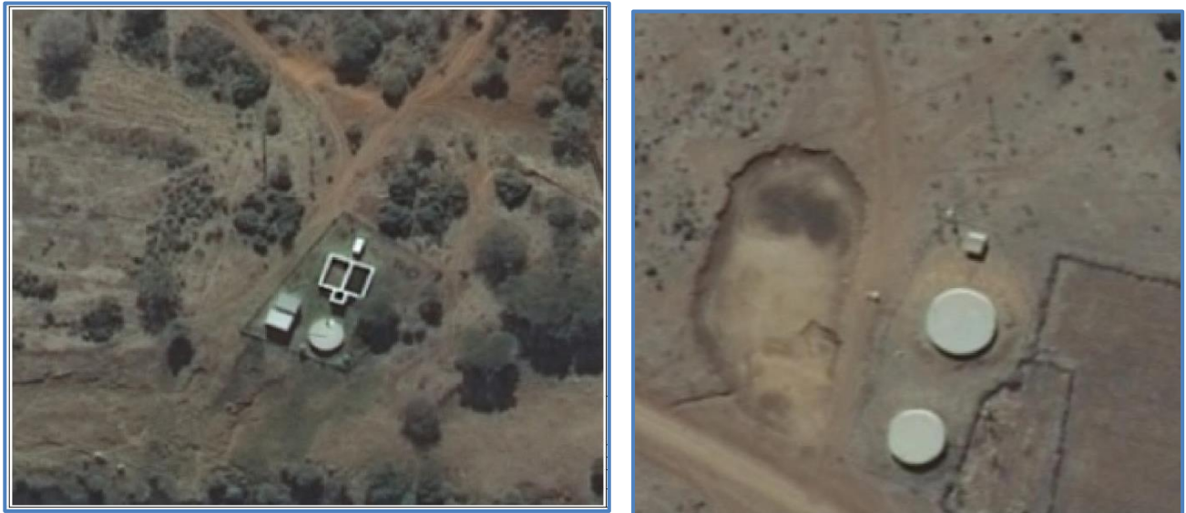
Figure 17.63 Aerial view of Nondebuya Water Treatment Plant & Nondabuya Reservoirs
