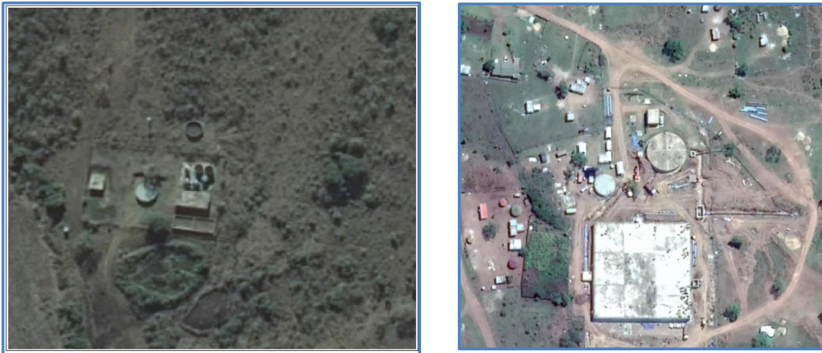
Figure 17.65 shows an aerial view of the Othobothini WTP
