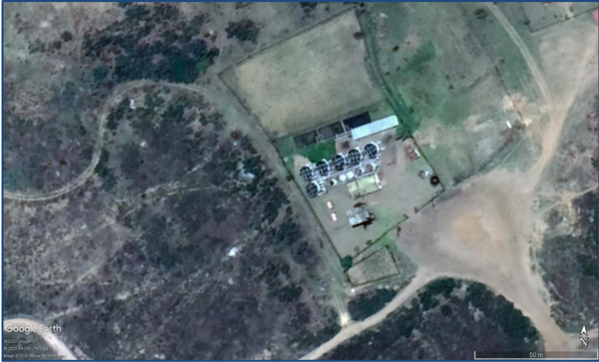
Figure 17.46 Aerial View of the Hlobane WTP
