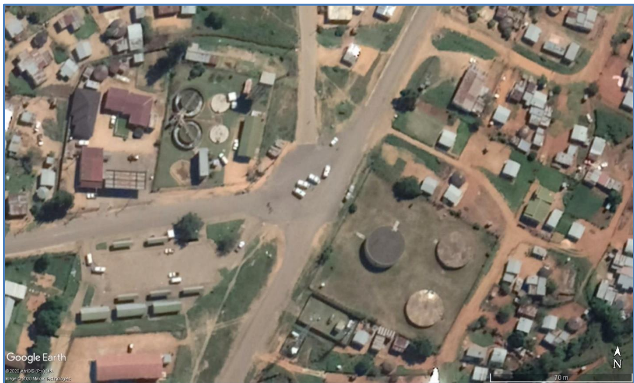
Figure 17.53 Aerial view of Frischgewaagd Water Treatment Plant
