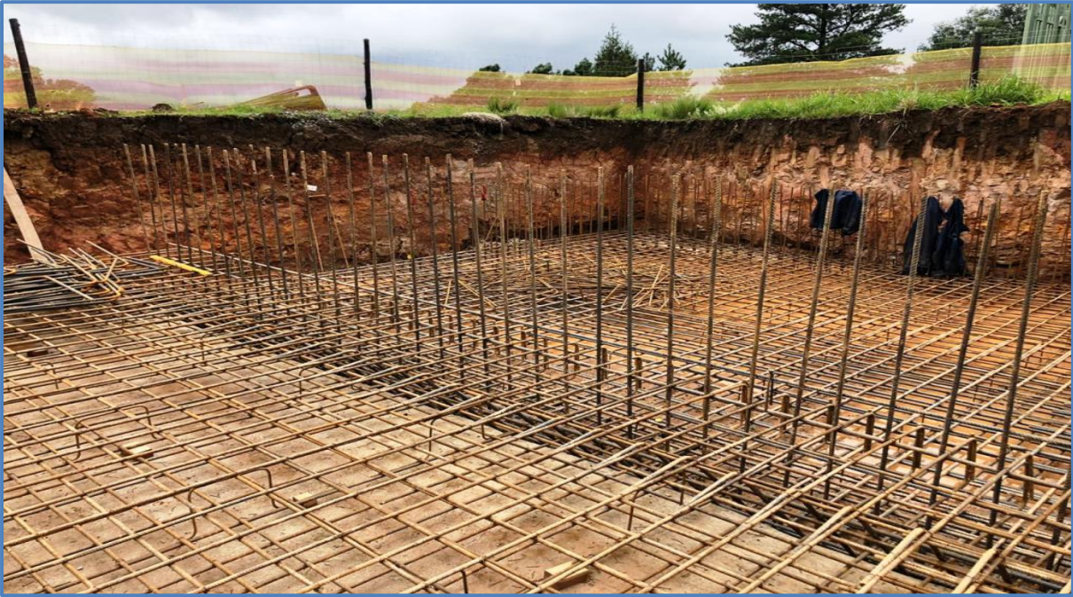
Figure.12.48 Transfer Pump Station in Construction (Late 2019)
