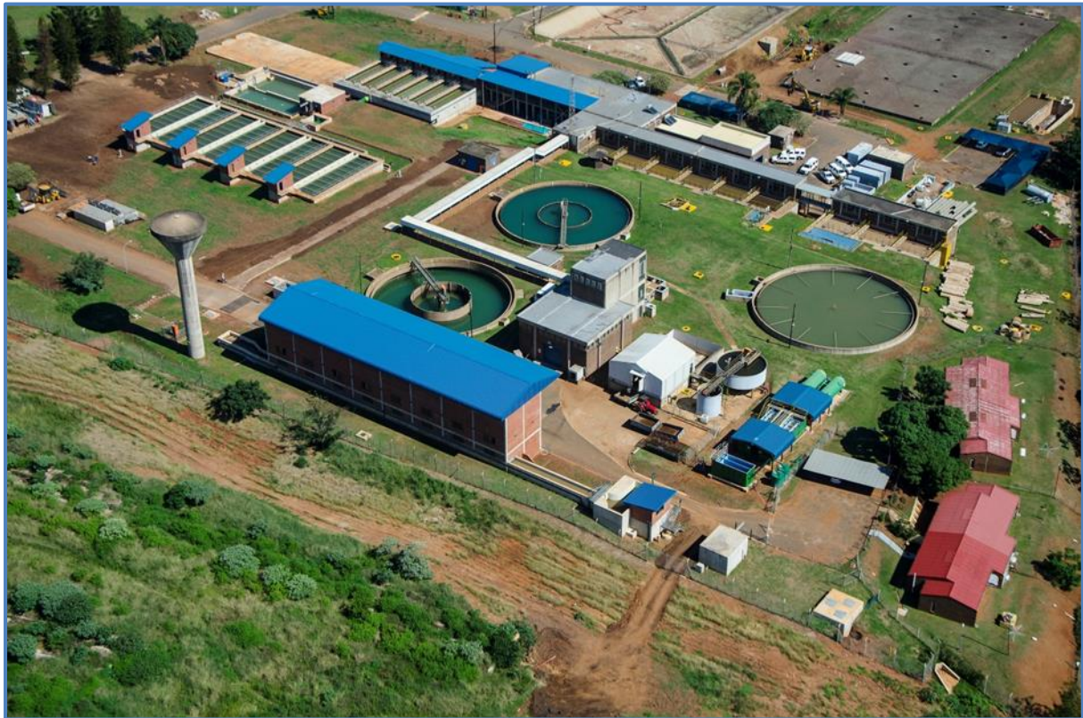
Figure 12.18 Hazelmere Water Treatment Plant.
