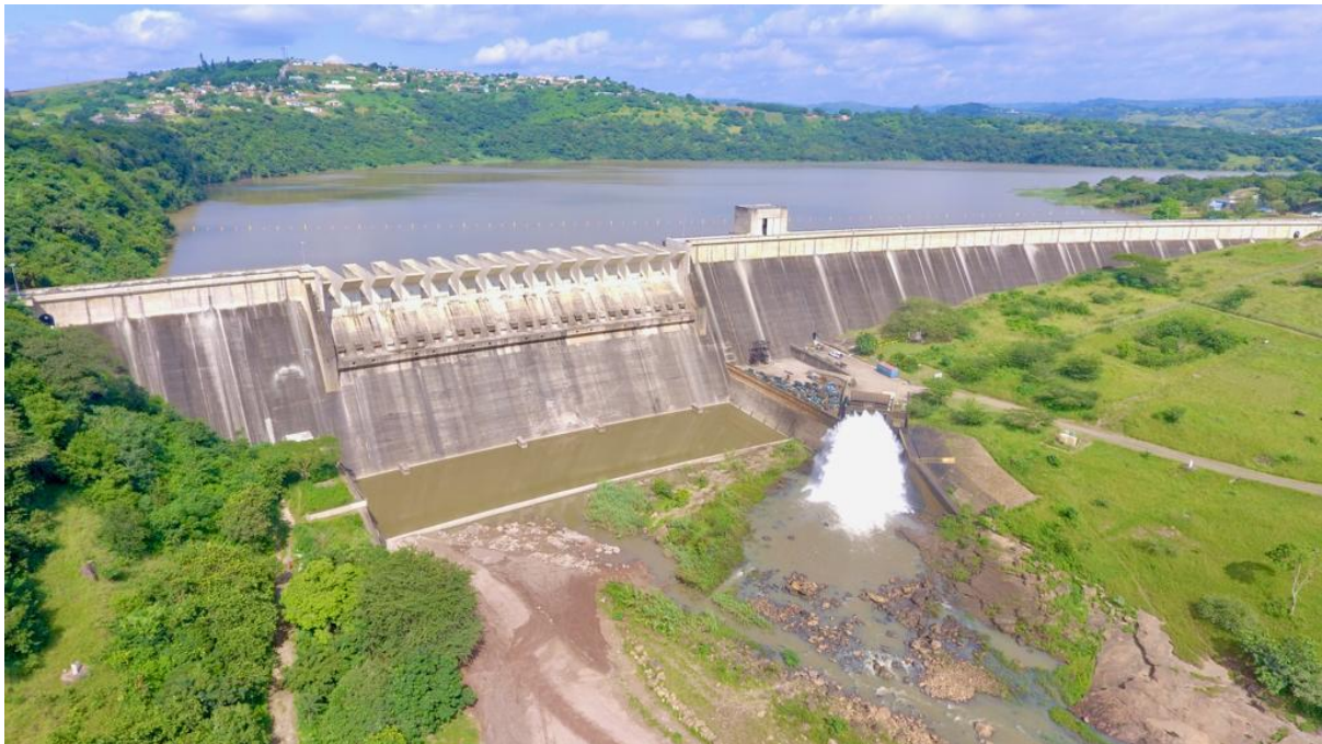
Figure 12.15 Hazelmere Dam showing raise dam wall.
