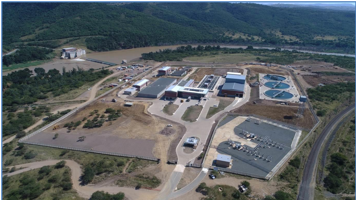
Figure 12.20 Lower Thukela Water Treatment Plant
