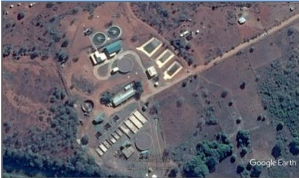
Figure 17.73 Aerial view of Shemula New Water Treatment Plant (Google Earth 2020: website).
