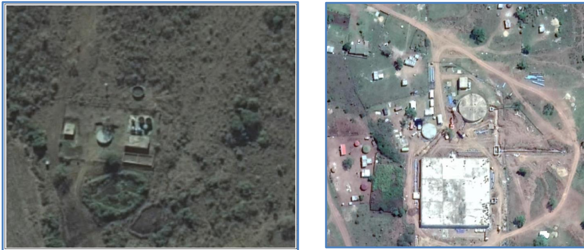
Figure 17.65 shows an aerial view of the Othobothini WTP (unknown source).
