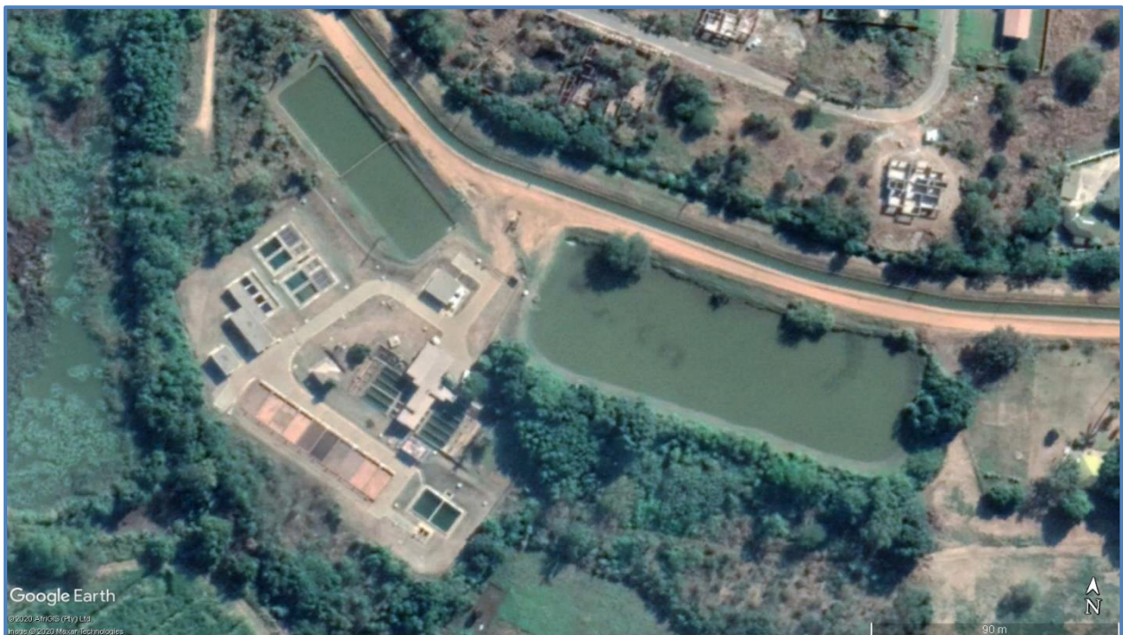
Figure 17.59 Aerial view of Phongola Water Treatment Plant
