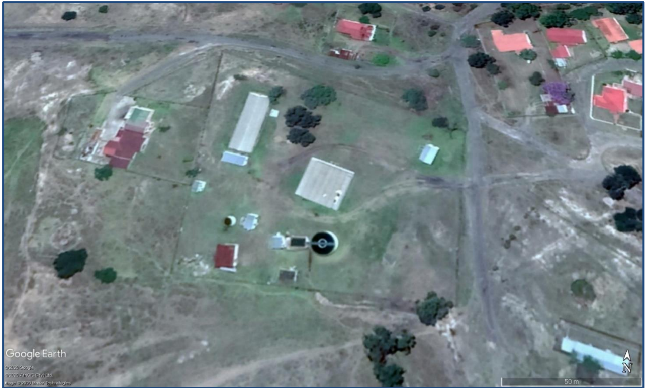
Figure 17.48 Aerial view of Coronation WTP (Google Earth 2020: website).
