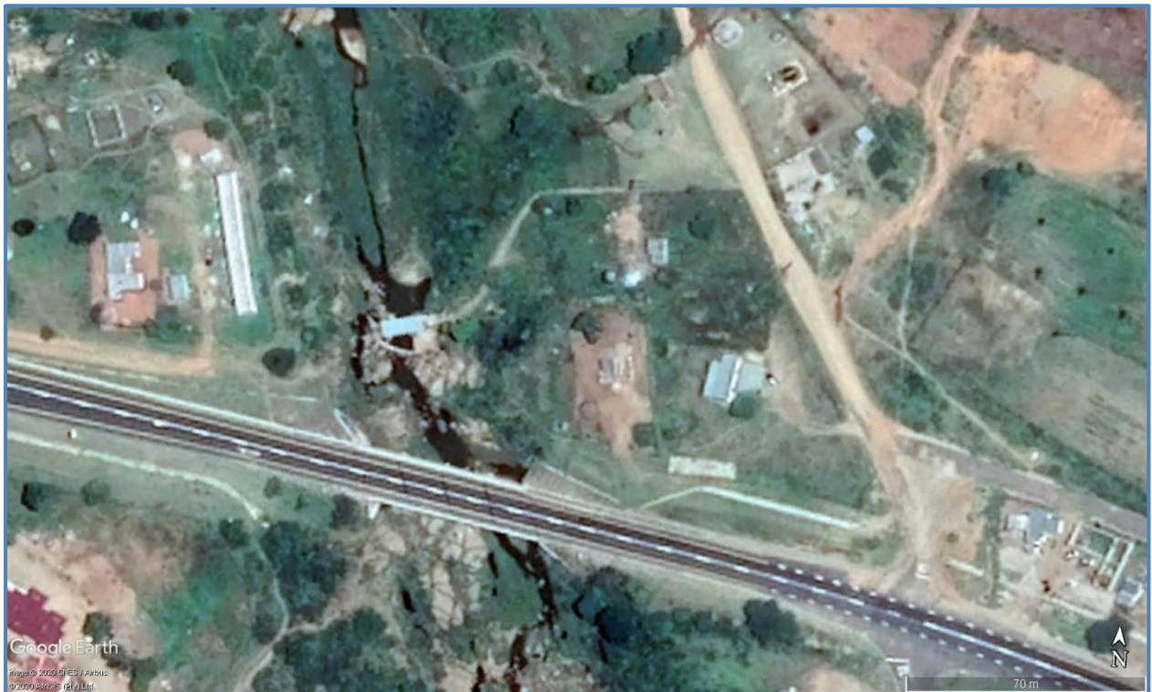
Figure 17.57 Aerial view of Spekboom Water Treatment Plant (Google Earth 2020: website).
