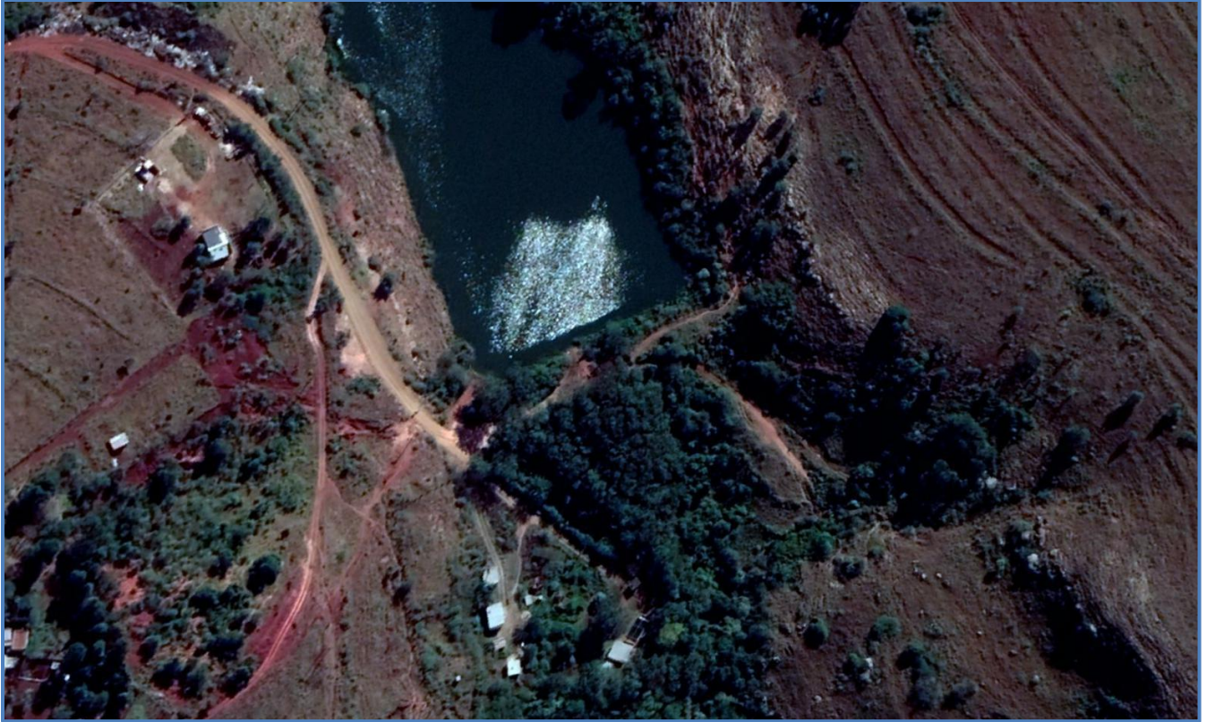
Figure 17.24 An Aerial view of the Embile WTP and the Embile Dam (Google Earth 2020: website).
