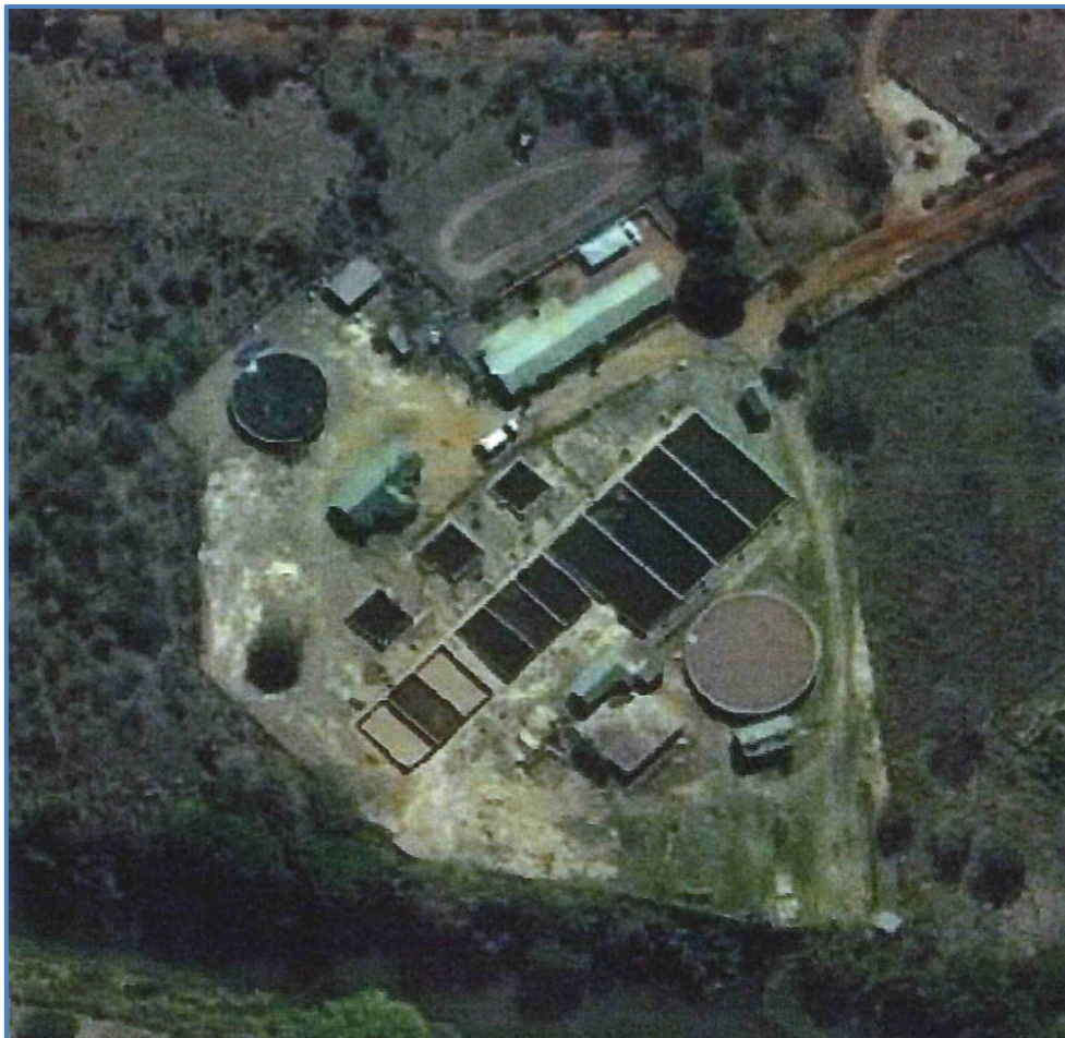
Figure 17.72 Aerial view of the Shemula (Old) WTP (unknown source).
