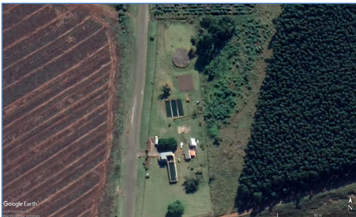
Figure 17.51 Aerial view of Edumbe Water Treatment Plant (Google Earth 2020: website).
