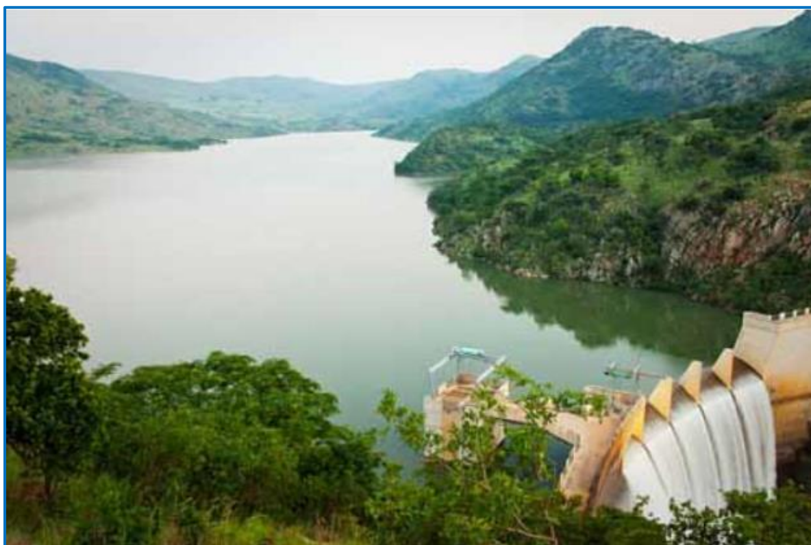
Figure 17.40 Bivane Dam - Source ( http://www.bestfishingspots.co.za/dam )
