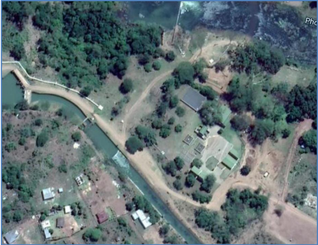
Figure 17.68 Aerial view of Jozini New Water Treatment Plant (unknown source).
