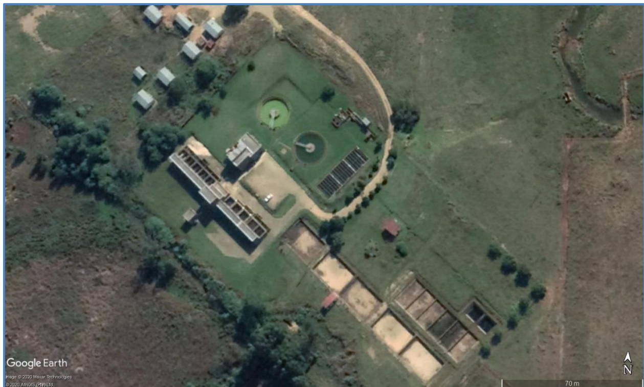
Figure 17.26 An Aerial view of the Bloemveld WTP (Google Earth 2020: website).
