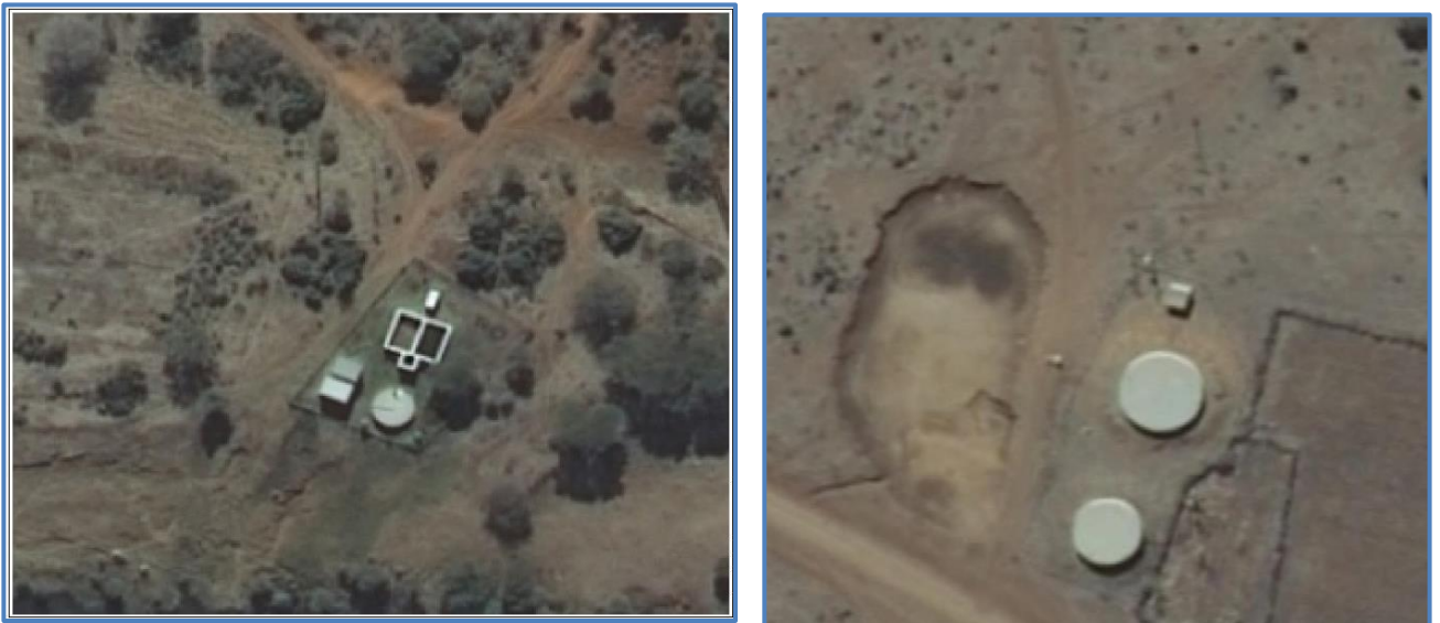
Figure 17.63 Aerial view of Nondebuya Water Treatment Plant & Nondabuya Reservoirs (unknown source).
