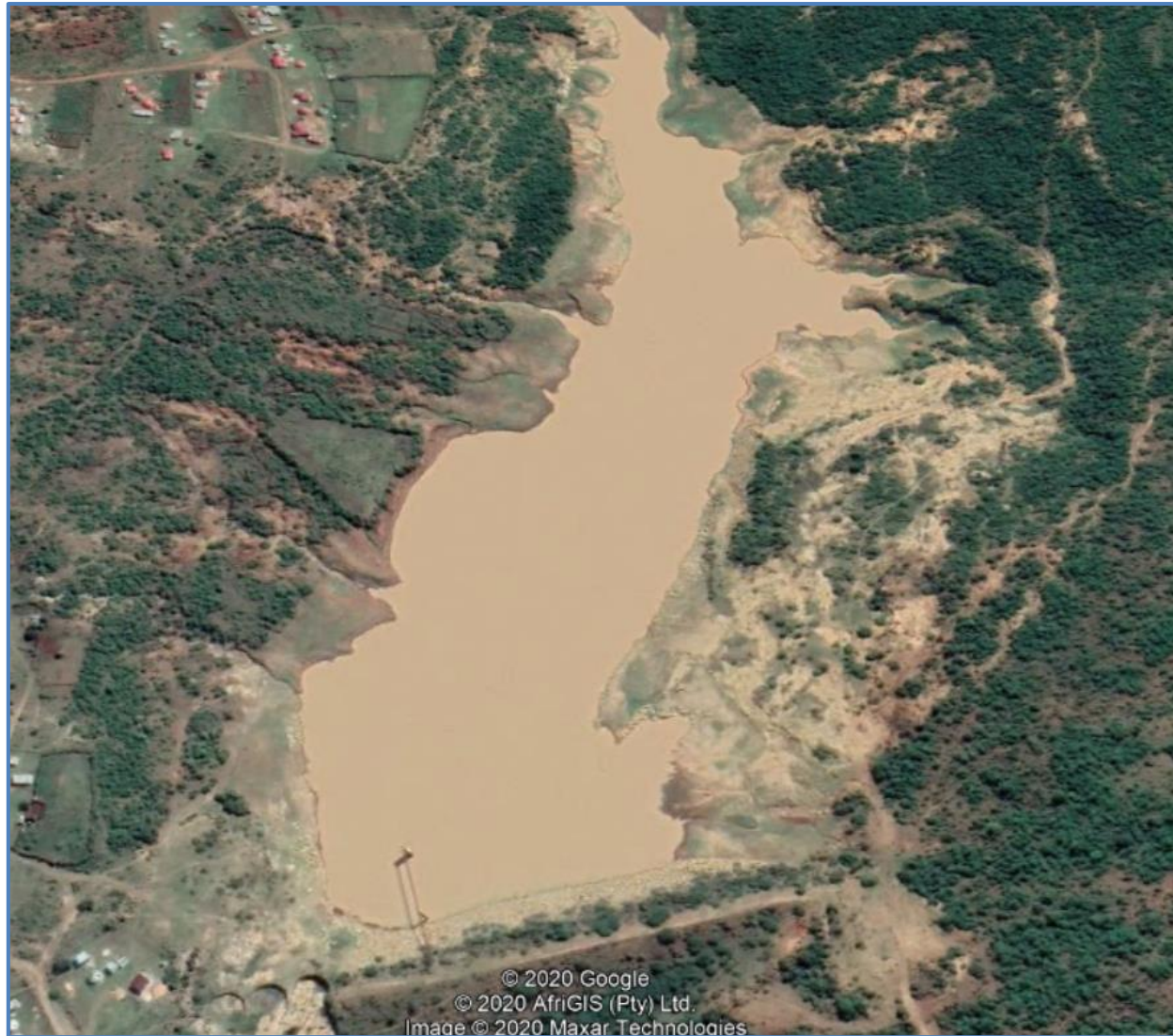
Figure 17.9 Vokwana Dam (Google Earth 2020)
