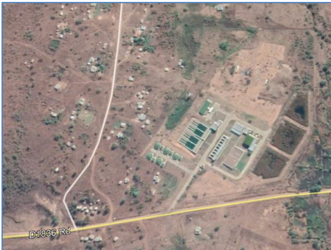
Figure 17.76 Aerial view of Regional Water Treatment Plant (NEW) (unknown source).
