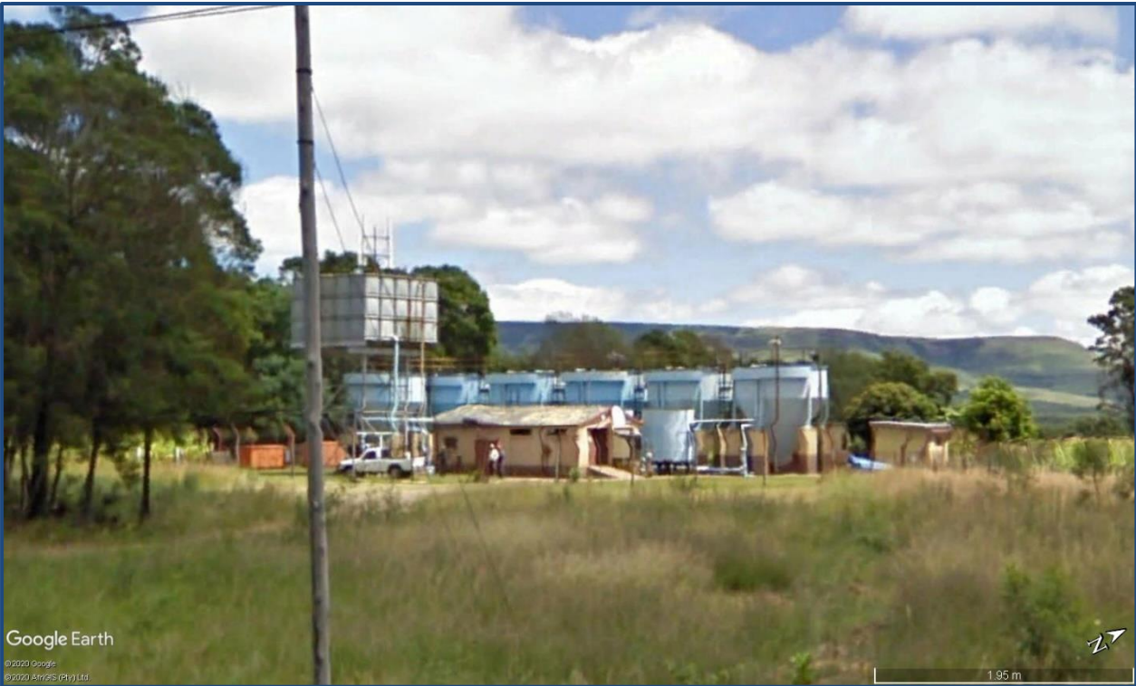
Figure 17.47 Hlobane WTP (Google Earth 2020: website).
