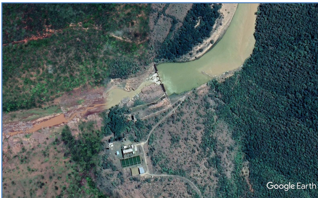
Figure 17.16 Aerial view of the weir and Ulundi Water Treatment Plant.
