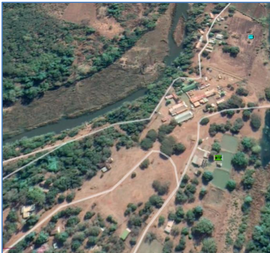
Figure 17.61 Aerial view of Mjindi Water Treatment Plant (Unknown source).
