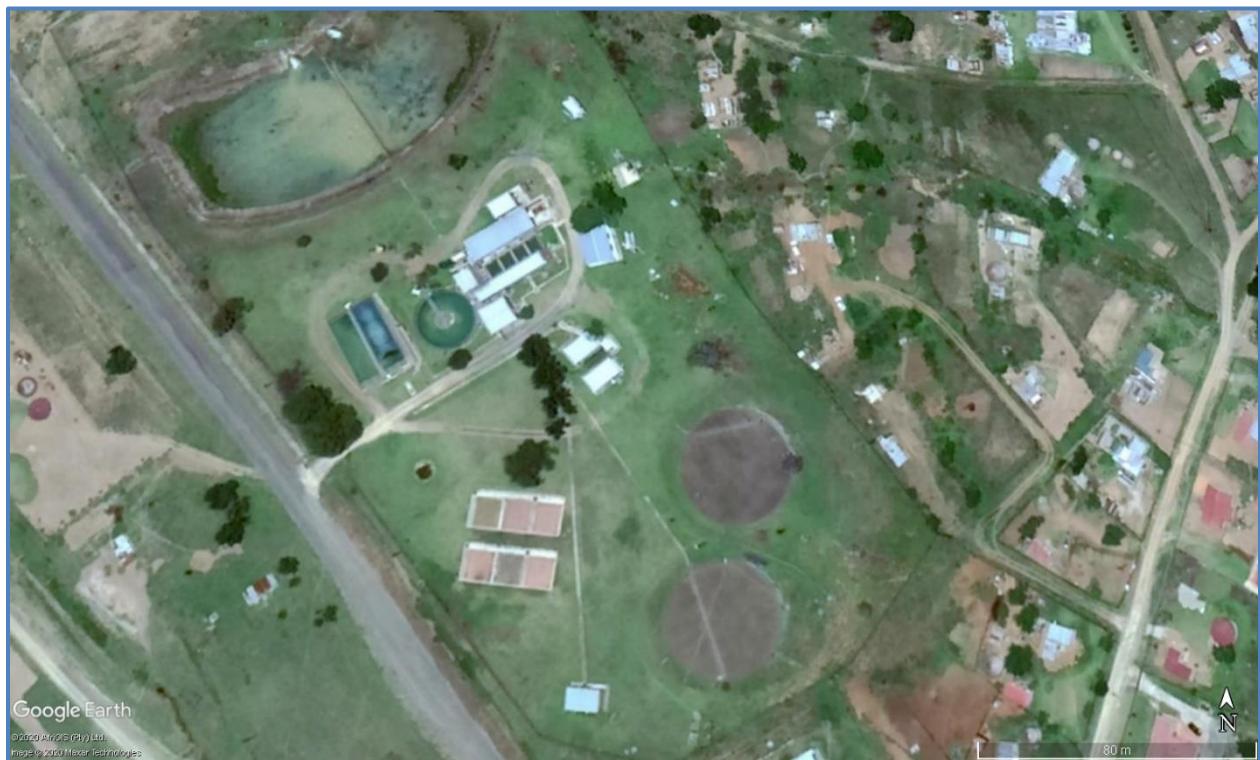
Figure 17.29 An Aerial view of the Mondlo WTP (Google Earth 2020: website).
