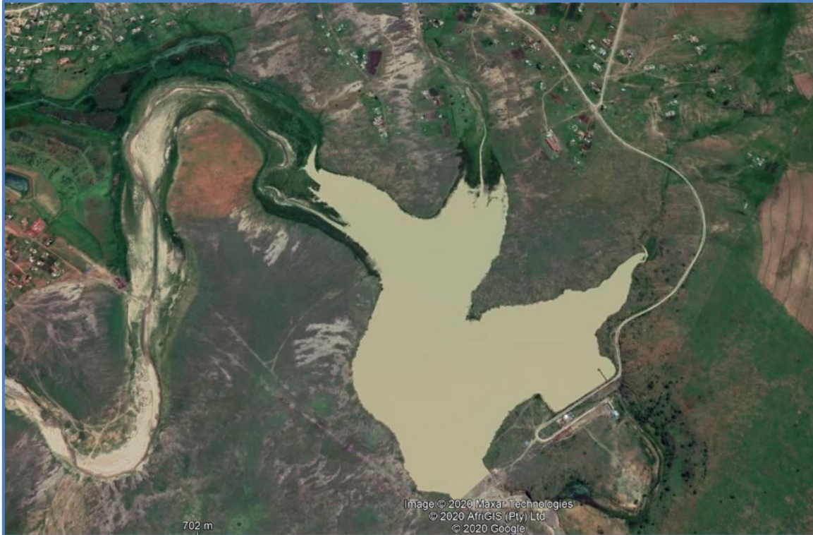
Figure 17.10 Mvunyana Dam (Google Earth 2020)
