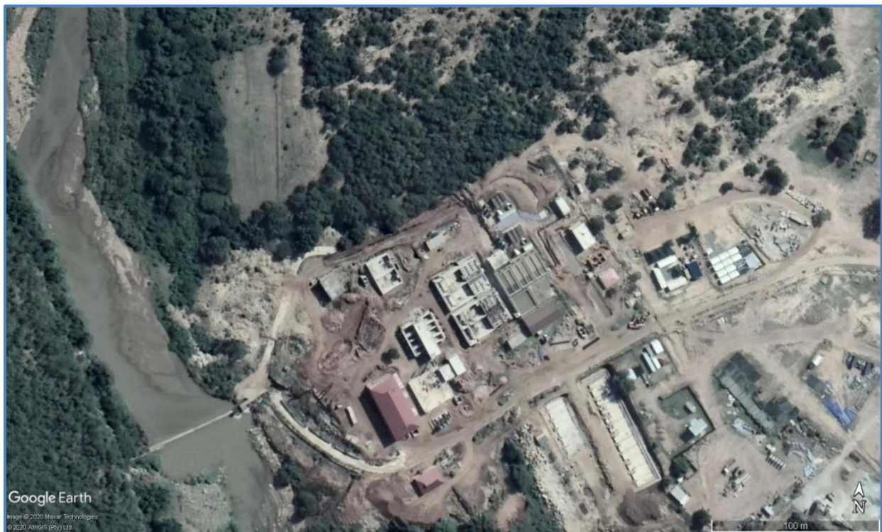
Figure 17.21 An Aerial view of the Usuthu WTP (Google Earth 2020: website).
